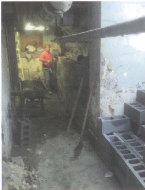
Photo 11 of 12 performance level 053.jpg Date: 05.10.2011 Basement - erecting new cinder block wall
