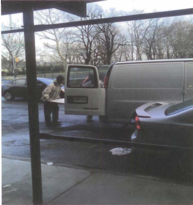
Photo 1 of 1 Inadequacies – dry wall being taken from building
