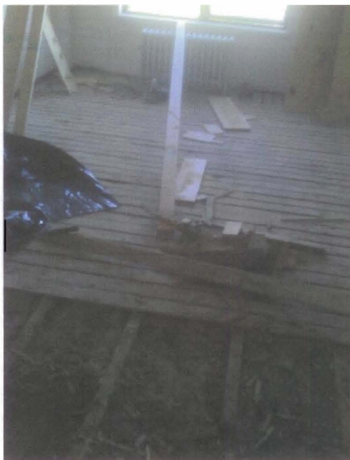
Photo 7 of 12 performance level 037.jpg Date: 05.10.2011 10F Living Rm. demolition of floor
