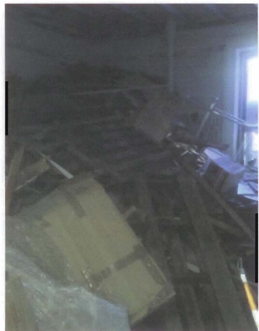
Photo 8 of 12 performance level 043.jpg Date: 05.10.2011 1F Living Rm. debris staging area
