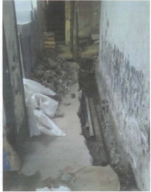
Photo 10 of 12 performance level 050.jpg Date: 05.10.2011 Basement - trenching for new pipes
