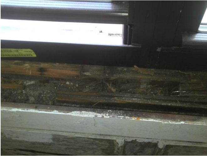
Photo 2 of 2 Inadequacies – dry wall being taken from building
