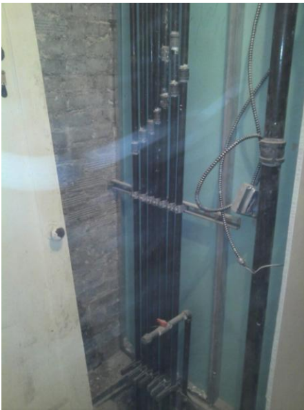
Photo 3 of 3 – Performance Level – 5F new gas lines
