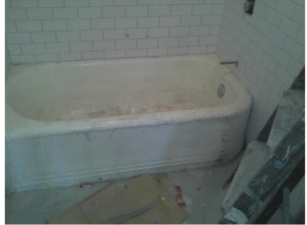
Photo 2 of 3 - Performance level – 4F bathroom
