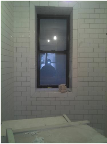
Photo 1 of 3 – Performance Level – 5F bathroom
