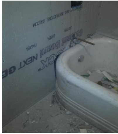
Photo 2 of 4 - Performance level - 1F bathroom
