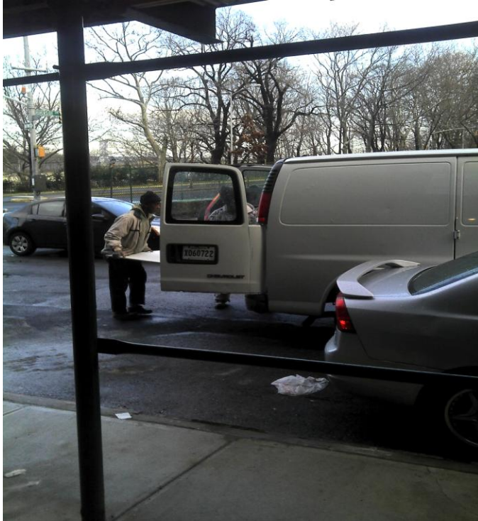
Photo 1 of 1 Inadequacies – dry wall being taken from building
