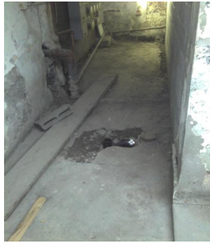
Photo 4 of 4 - Performance Level - basement drain
