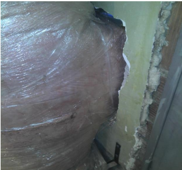
Photo 3 of 5 performance level Date: 11-3-2011 7F trash chute
