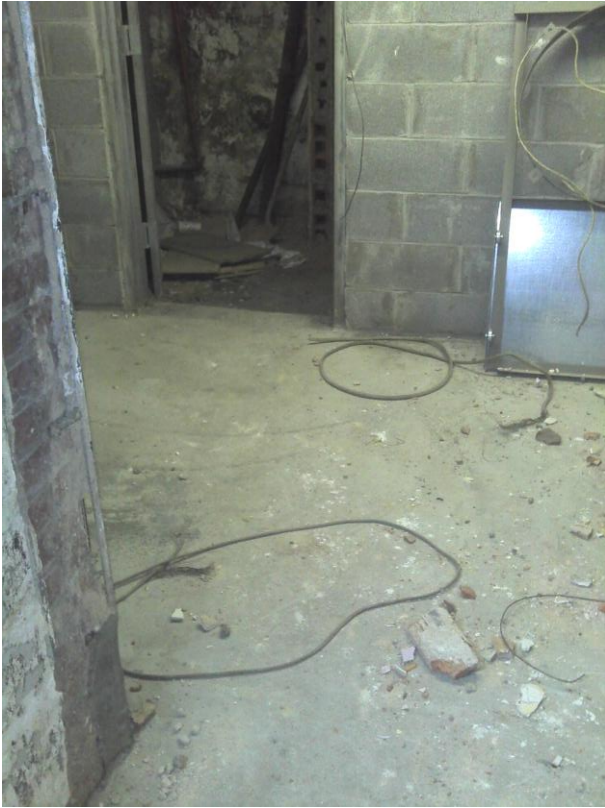
Photo 3 of 5 performance level Date: 11-3-2011 Basement - new concrete floor
