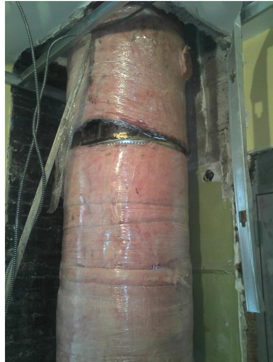
Photo 2 of 5 performance level Date: 11-3-2011 11F trash chute
