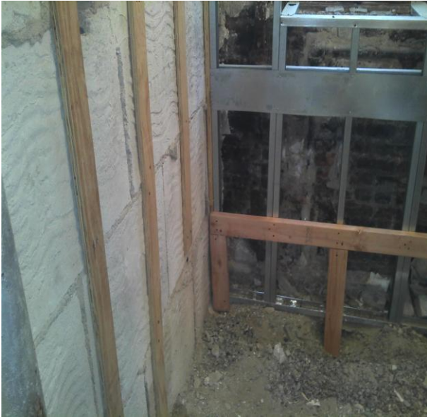
Photo 1 of 5 performance level Date: 11-3-2011 11F wall furring
