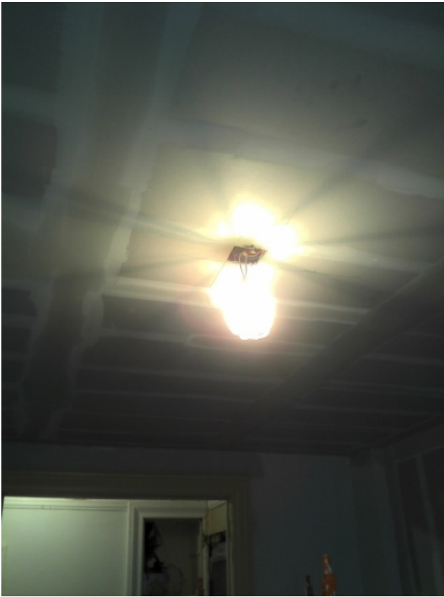
Photo 7 of 11 performance level 022.jpg Date: 17.11.2011 8F ceiling living room
