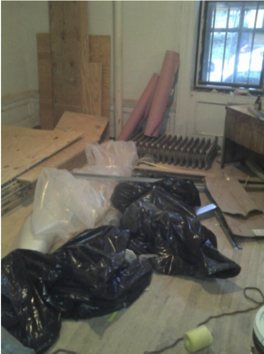
Photo 1 of 11 performance level 001.jpg Date: 17.11.2011 1F staging apartment
