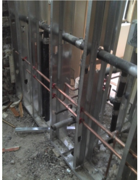
Photo 2 of 11 performance level 011.jpg Date: 17.11.2011 12F bathroom - plumbing and framing.
