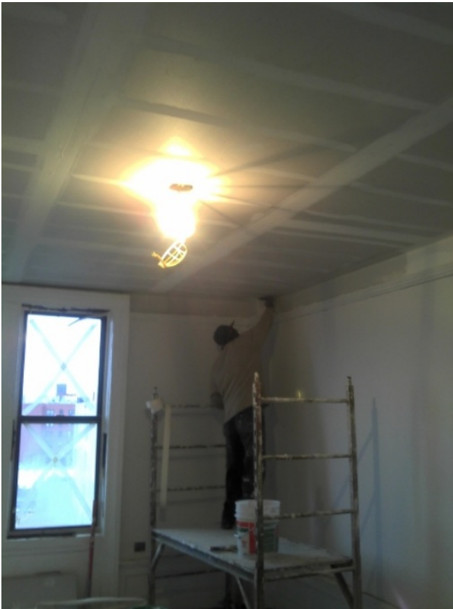
Photo 5 of 11 performance level 015.jpg Date: 17.11.2011 12F patching drywall
