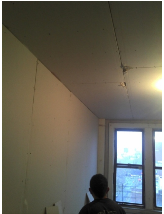
Photo 8 of 11 performance level 033.jpg Date: 17.11.2011 7F installing drywall (sheet rock)
