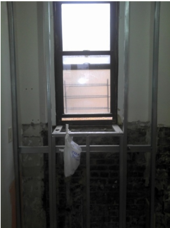
Photo 3 of 11 performance level 012.jpg Date: 17.11.2011 12F framing of window in bathroom
