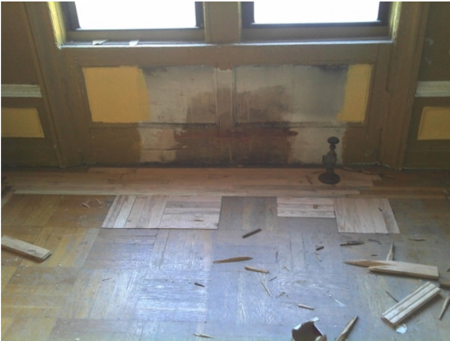
Photo 8 of 9 performance level 080.jpg Date: 17.10.2011 4F selective replacement flooring
