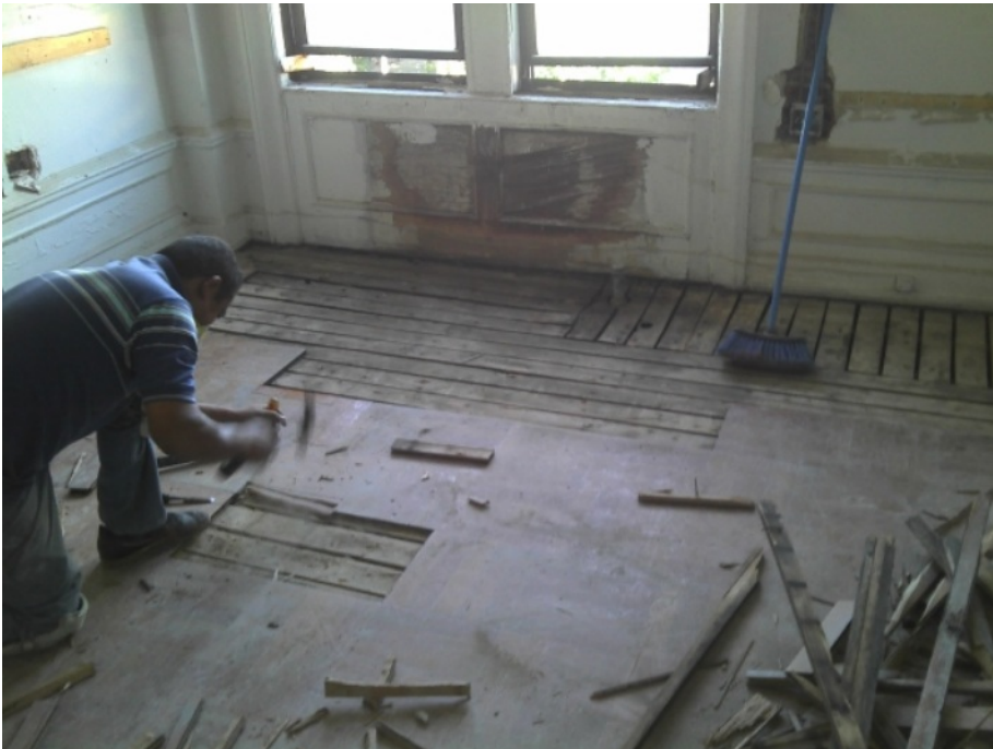
Photo 7 of 9 performance level 077.jpg Date: 17.10.2011 5F flooring work
