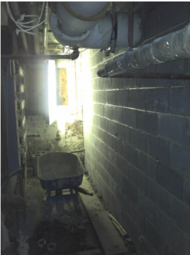
Photo 9 of 9 performance level 093.jpg Date: 17.10.2011 Cinder block wall complete in basement
