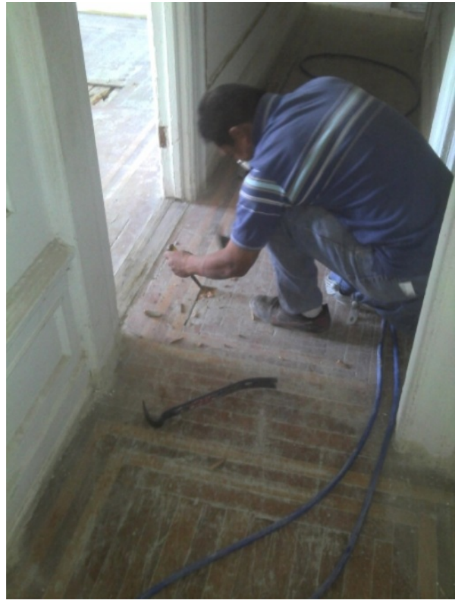
Photo 6 of 9 performance level 033.jpg Date: 17.10.2011 5F flooring work
