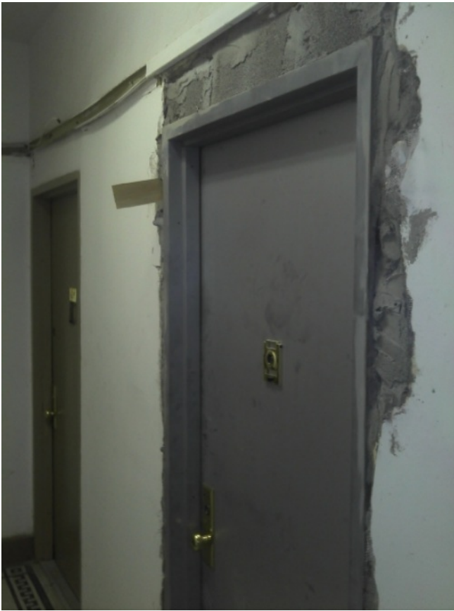
Photo 5 of 9 performance level 031.jpg Date: 17.10.2011 7F second means of egress installed
