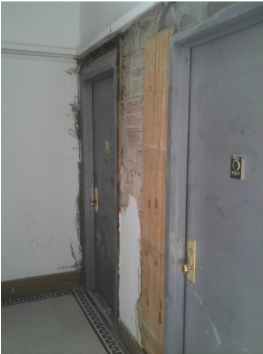
Photo 1 of 9 performance level 004.jpg Date: 17.10.2011 New Doors and hardware installed 12F
