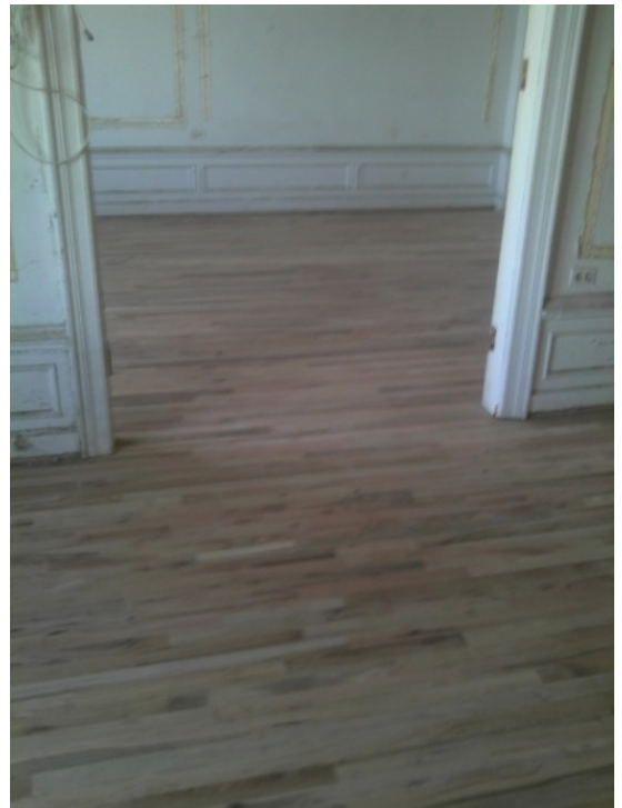
Photo 4 of 9 performance level 019.jpg Date: 17.10.2011 10F Flooring
