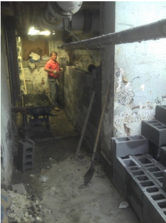
Photo 11 of 12 performance level 053.jpg Date: 05.10.2011 Basement - erecting new cinder block wall
