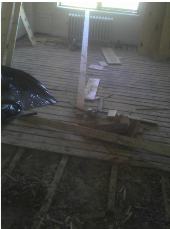
Photo 7 of 12 performance level 037.jpg Date: 05.10.2011 10F Living Rm. demolition of floor
