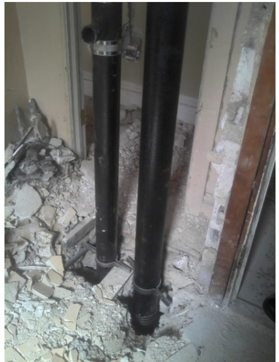
Photo 4 of 12 performance level 010.jpg Date: 05.10.2011 12F Bathroom new galvanized pipes
