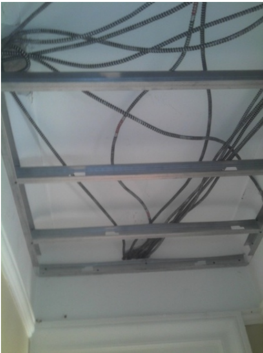
Photo 3 of 12 performance level 007.jpg Date: 05.10.2011 12F Hallway wiring ceiling
