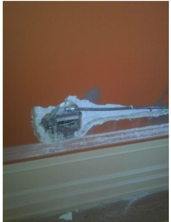
Photo 2 of 12 performance level 005.jpg Date: 05.10.2011 12F - Living Rm. wall wiring
