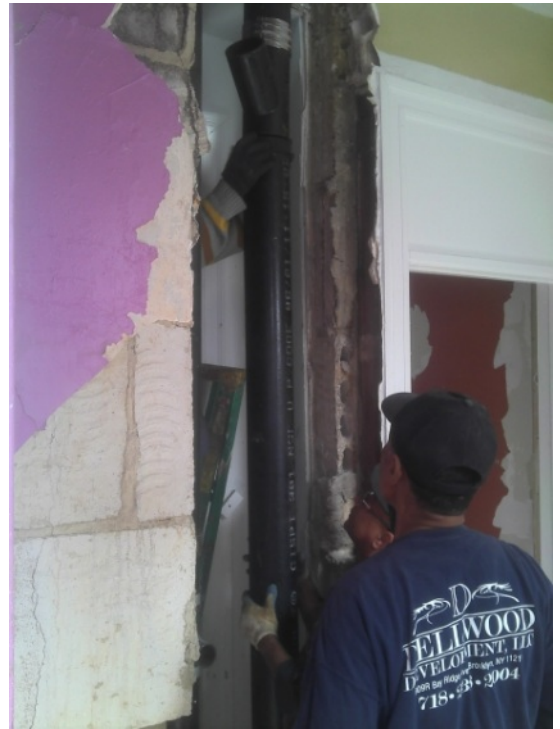
Photo 6 of 12 performance level 036.jpg Date: 05.10.2011 11F Bathroom installation of new pipes
