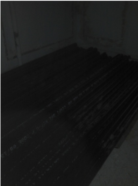
Photo 9 of 12 performance level 047.jpg Date: 05.10.2011 1F Bedroom - new pipe staging area
