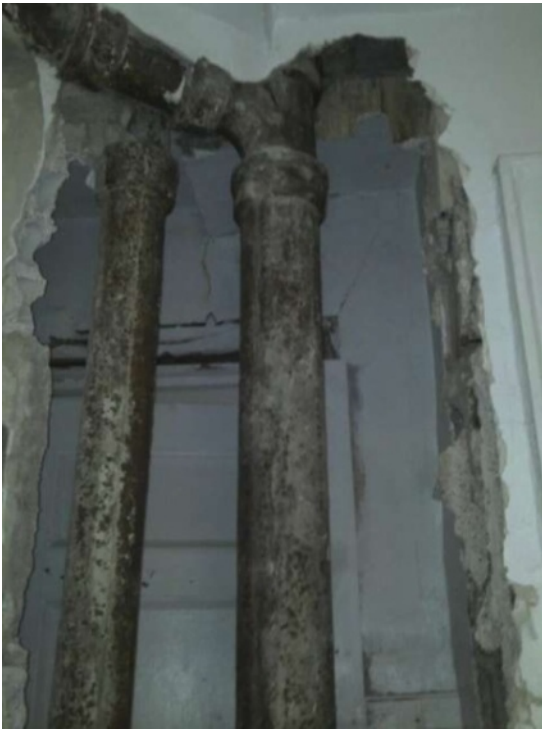
Photo 6 of 5 performance level 035.jpg Date: 14.09.2011 8F waste line
