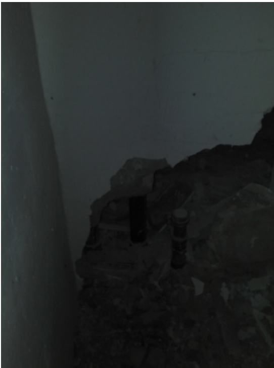
Photo 4 of 5 performance level 045.jpg Date: 14.09.2011 8F water domestic off chaise in water closet
