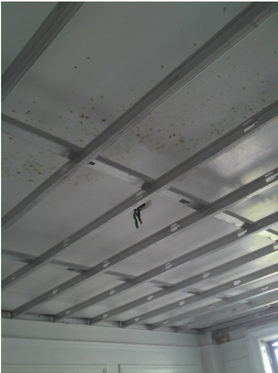
Photo 1 of 5 performance level 040.jpg Date: 14.09.2011 11F ceiling frame
