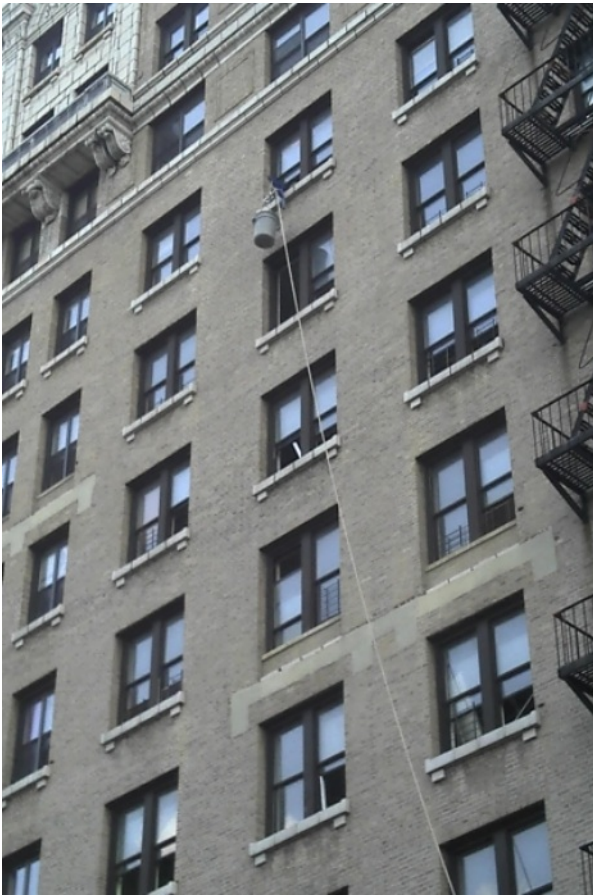
Photo 1 of 4 performance level 002.jpg Date: 13.09.2011 Bucket with pulley from 7th floor
