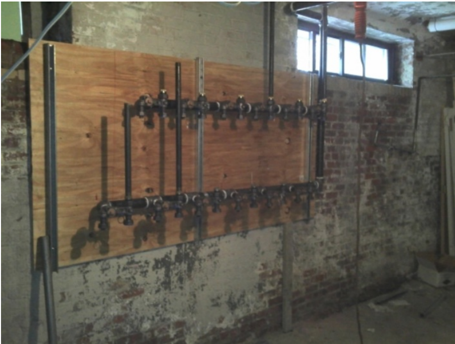
Photo 3 of 4 performance level 030.jpg Date: 13.09.2011 Gas meter roughing in basement
