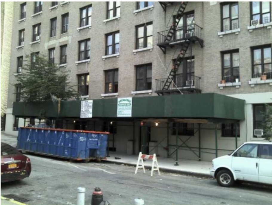
Photo 1 of 4 inadequacies 004.jpg Date: 13.09.2011 Scaffolding - location different from last visit
