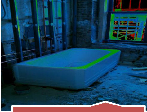
Performance level: Set tub, furred out wall and unfinished floor (4G)
