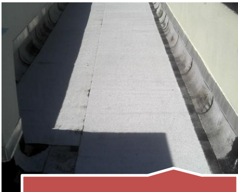
Performance Level: Counter flashing above roof surface cap.
