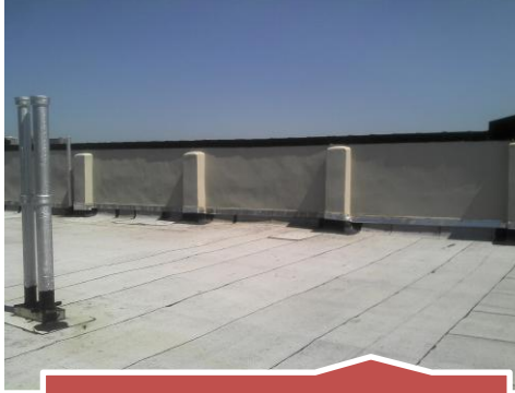
Performance Level: Roof and parapet wall
