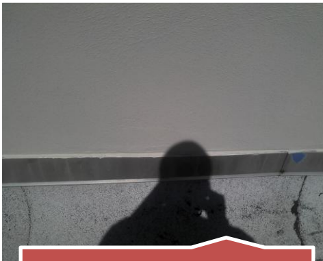
Performance Level: Counter flashing above roof surface cap.
