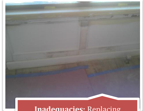
Inadequacies: Replacing damaged wall panel behind former radiators.
