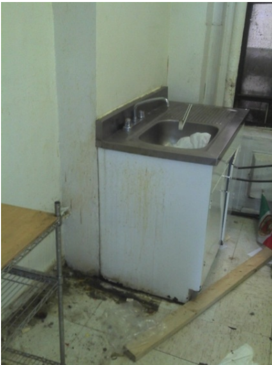
Photo 3 of 4 performance level 002.jpg Date: 17.08.2011 5th Floor F - Kitchen
