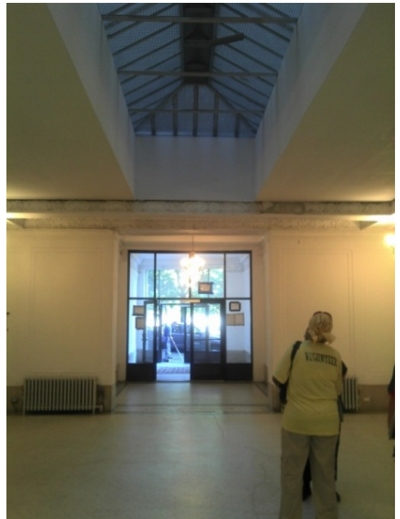
Photo 4 of 4 performance level 004.jpg Date: 17.08.2011 Entrance - Common Area 1st floor
